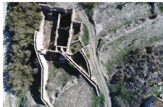
Catalans Factory. Current aerial view.
